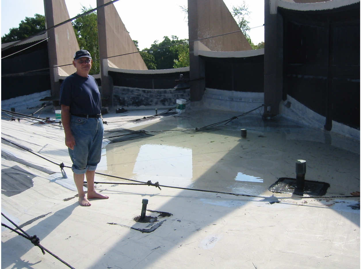
Ponding on the roof continued to be a problem because the drains needed to be improved and debris removal, freezing within, and such matters needed to be prevented. Here Stu prepares to enter the lake and open one of four drains. This particular drain was relined with hose to prevent the leak inside Servetus (October, 2005).
