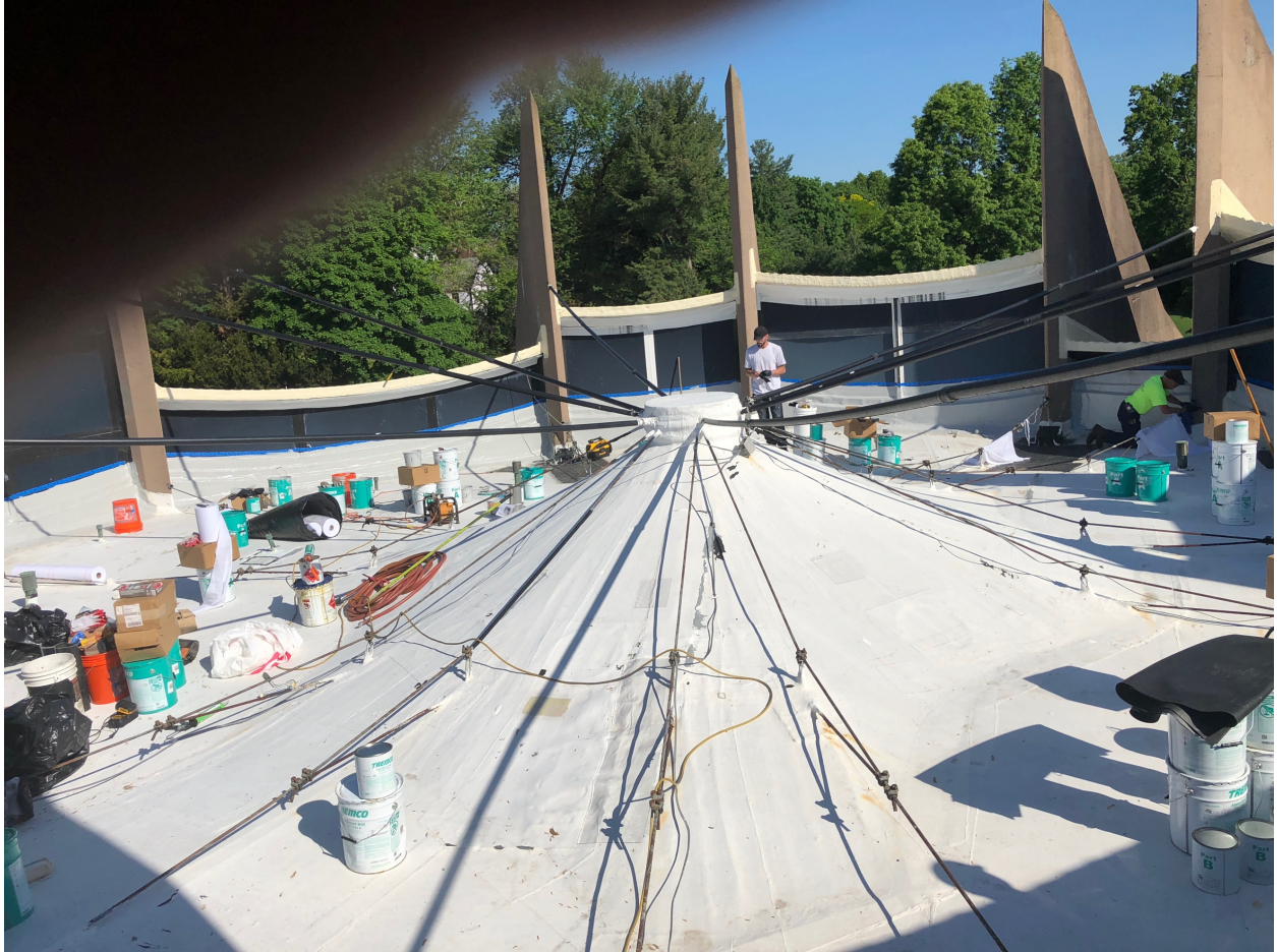
In 2018 a new methodology was employed to repair, recover and improve the roof. Here the contractor is surrounded by buckets of fluids and equipment used to apply a new tough membrane covering the entire roof (May 2018).
